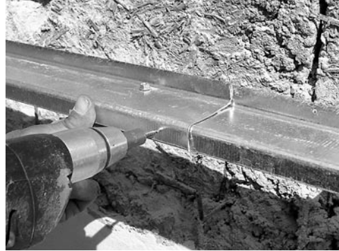
Connection of Z50 profiles, overlap 100 mm
